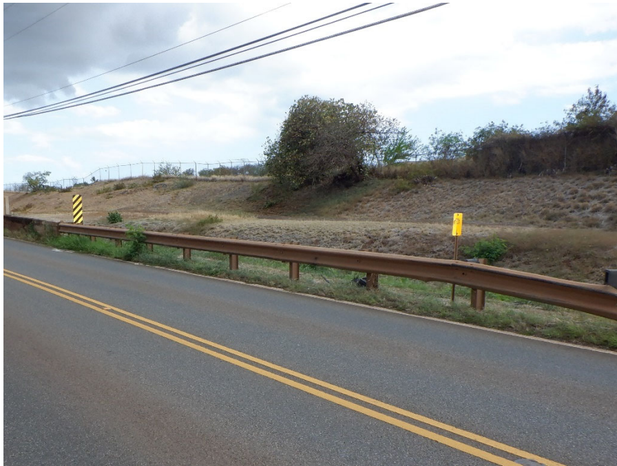
PHOTO 6 UPSTREAM NORTH APPROACH GUARDRAIL
