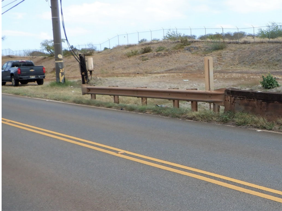
PHOTO 5 UPSTREAM SOUTH APPROACH GUARDRAIL
