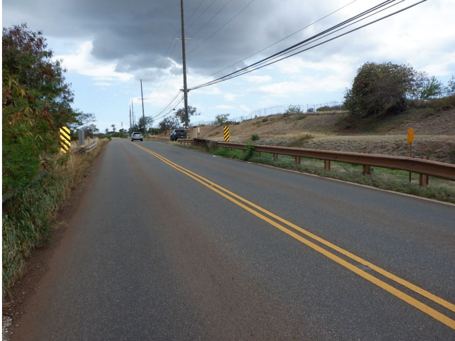
PHOTO 1 NORTH APPROACH LOOKING SOUTH
