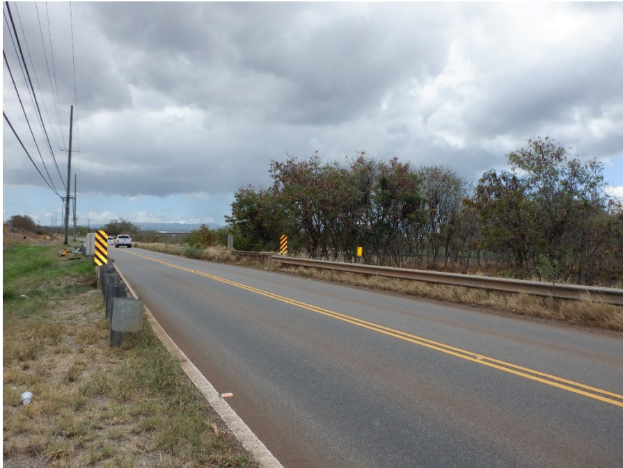
PHOTO 2 SOUTH APPROACH LOOKING NORTH
