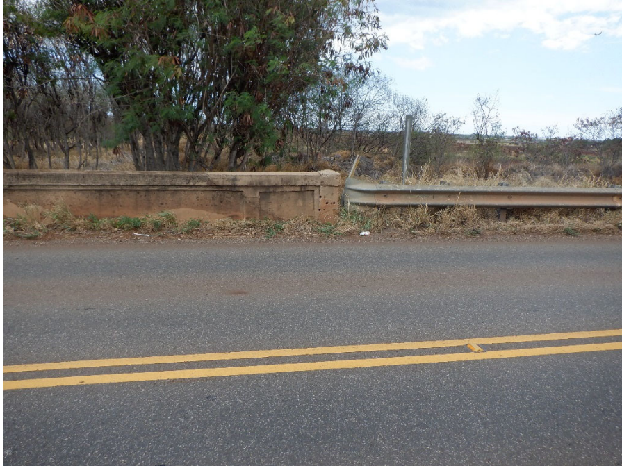
PHOTO 7 DOWNSTREAM SOUTH APPROACH GUARDRAIL
